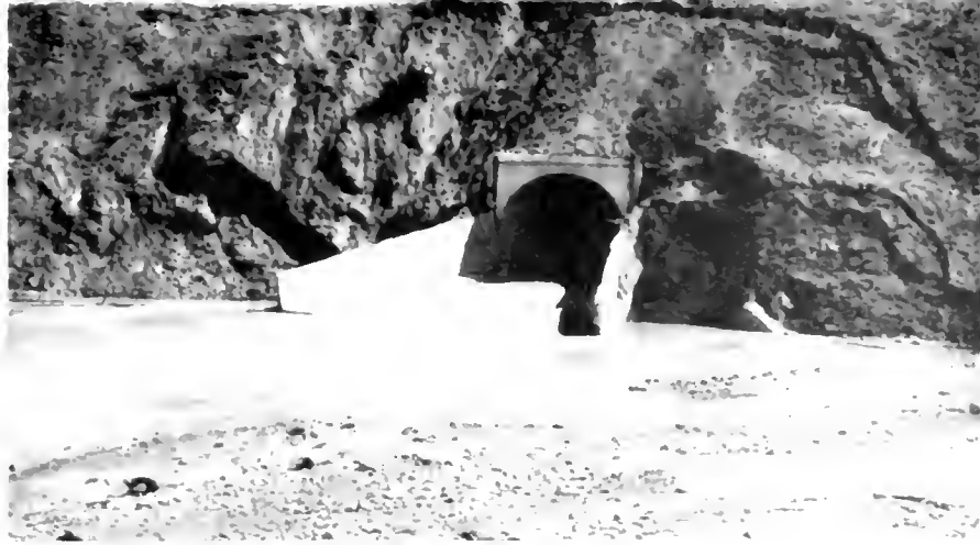
FIG. 33a. Nojoqui Creek culvert in 1940, after discharge of 640 second-feet
